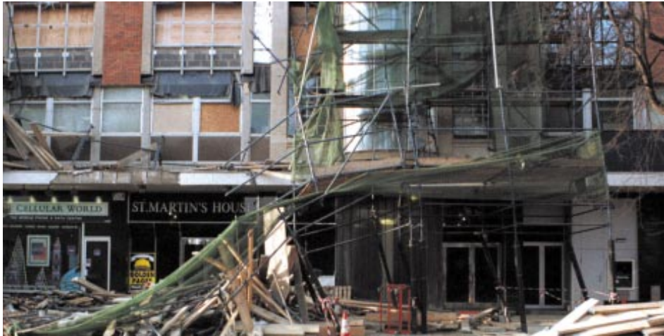
Accident scene in Dublin where three workmen were injured when scaffolding collapsed.
